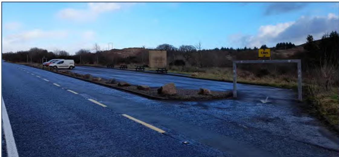
Plate 13-10 View from the west, approximately 1.1km from the onsite 110kV substation on the N15 National Road
