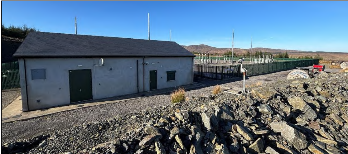
Plate 13-6 View facing northwest towards the onsite 110kV substation
